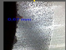
Flaking on the liner
